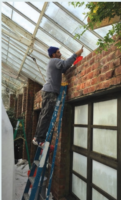
Crew from Mt. Olympus Restoration, Inc. restoring interior steel frame supports.
