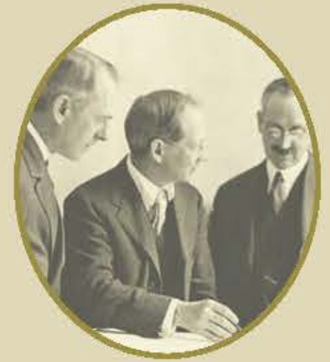
Courtesy of the United States Department of the Interior, National Park Service, Frederick Law Olmsted National Historic Site
